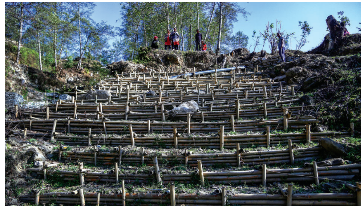
Community-centric landslide mitigation via nature-based solutions in Bhotenamlang, Sindhupalchok
