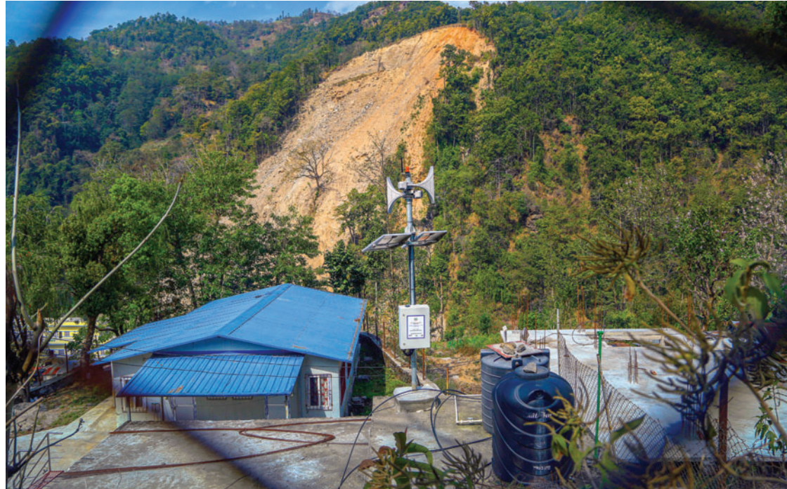
Emergency automatic siren for risk communication in Panchpokhari Thangpal, Sindhupalchok
